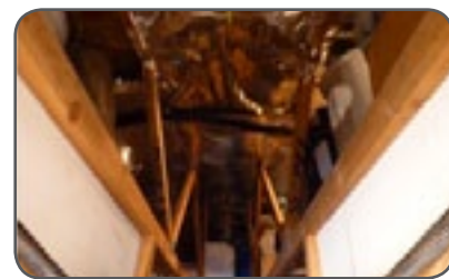
Radiant barrier in attic
